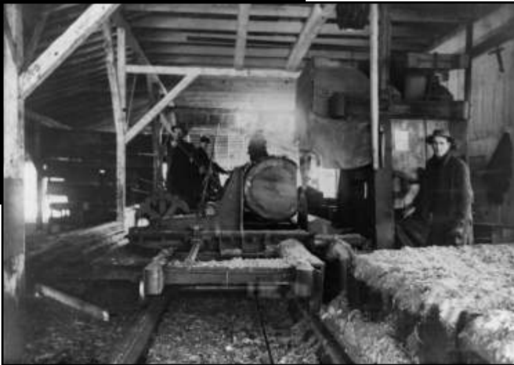
Figure 6: The inside of the Washington Mill/Standard Lumber Mill sometime in the first decade of the 20 th century. Note the two circular saws that cut the lumber from the log. Ernest DeVoe is the sawyer and Billy Mix and John Hickey are on the carriage. (Lawrence Zimmerer Photographic Collection)
