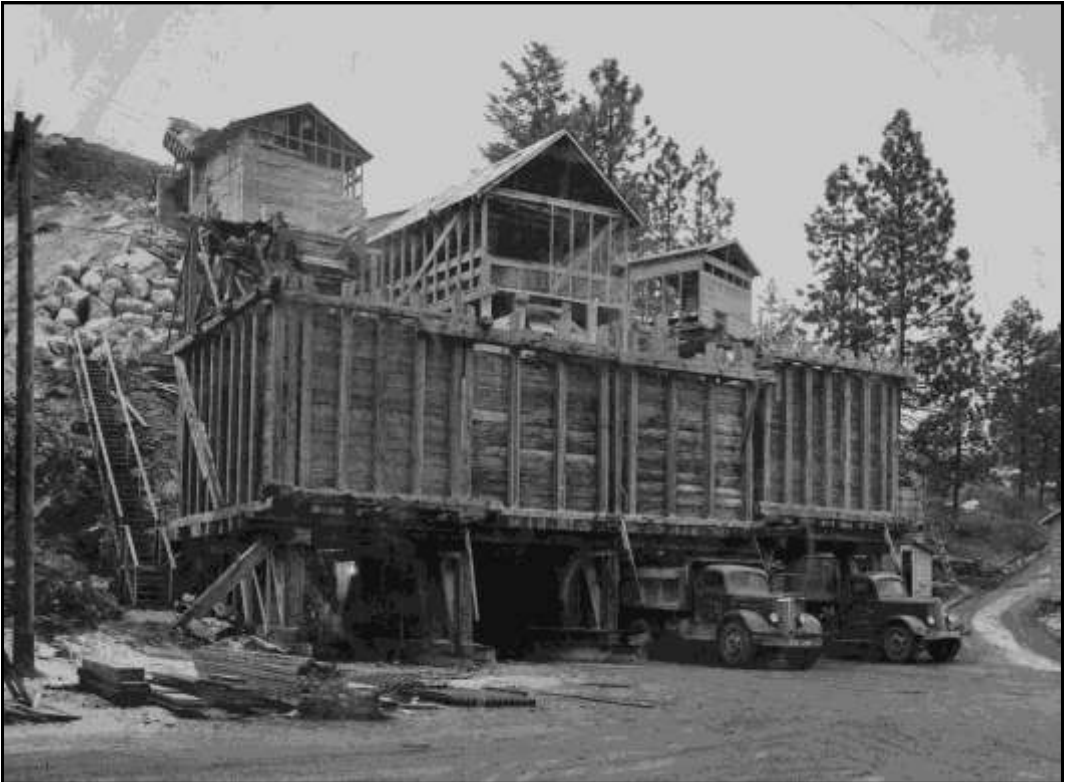
Figure 5: The crusher building is at the top of the picture where an elevated dump truck bed can be seen dumping ore into the crusher. The open framed buildings contained the vibrating screens that sorted the ore. The bunker at the far left held the finer material, bunkers to the right held increasingly coarse ore. The long handle at the right side of the base of the bunkers was the lever to open the bunker to the trucks below. The pit is over the hill in the background. (Melvin Mullenix Photograph)
