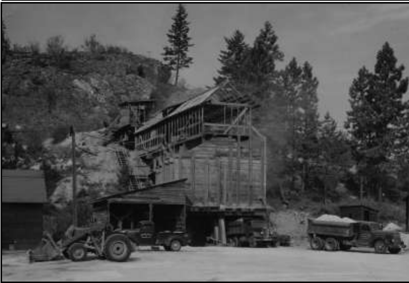
Figure 2: The two bay bunkers may have been built either by the National Chemical and Lime Company or the Gladding McBean Company in the late 1920s or 1930s. This picture was taken in the early 1940s. (Melvin Mullenix Photograph)
