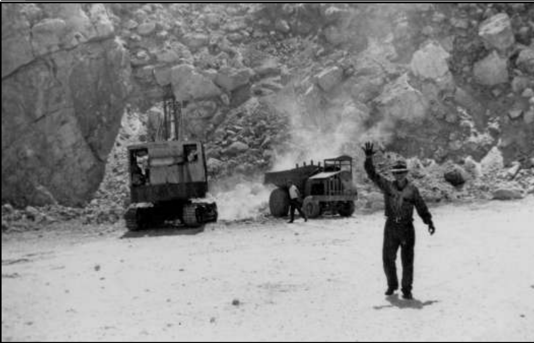
Figure 4: Shovel loading operations in the pit after the wall rock had been loosened by dynamite. (Melvin Mullenix Photograph)
