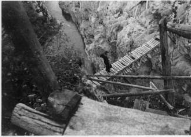
Bridge across Z canyon, photo ca 1939
