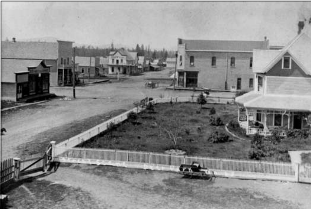
Photograph 2: West along Crawford Street across Main Avenue prior to 1908. This picture is prominently reproduced on the wall in Yoke’s Grocery Store on South Main Avenue. (Lawrence Zimmerer Photograph Collection)
