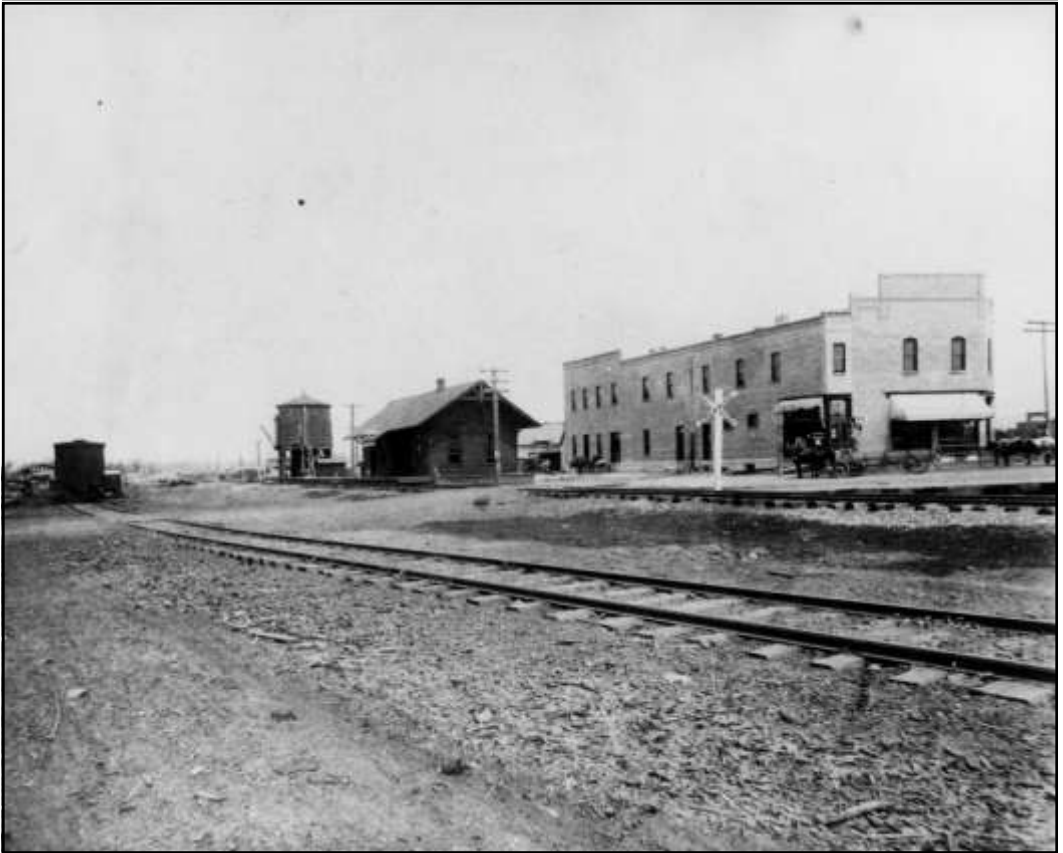
Photograph 3: The Kelly Store with the railroad tracks, station and water tower just west across Railroad Avenue about 1908. Note that the railroad rails have no tie plates with the rails spiked directly to the ties. (Lawrence Zimmerer Photograph Collection)
