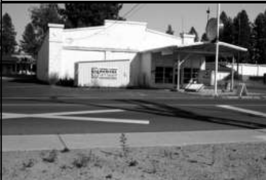
Photograph 10: The Deer Park Motor Company Garage building in August of 2009. This building had been a automobile repair shop for years until recently when it became a second hand shop. (Peter Coffin Photograph)
