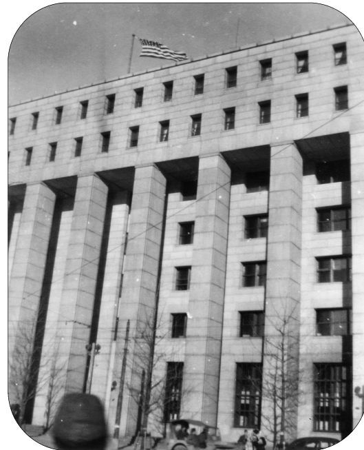
The Dai Ichi building; General Headquarters for the occupation. Dai Ichi means "number one" or "the first" in Japanese. It had been a bank.
