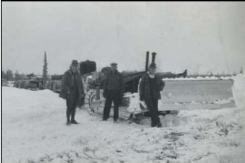
Figure 4: Hauling supplies to the mining area in 1937. Three to six feet of snow on the mountain in the winter months was not unusual. From the left Foster, Kimmel, A. W. Kemp. (Photograph from the Al Kemp Collec-
