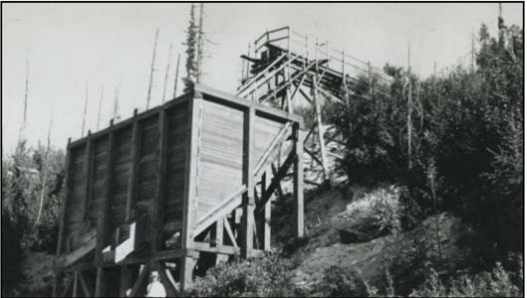
Figure 6: Ore bunker on Blue Grouse Mountain. Other pictures in the Kemp collection indicate that the mill is at the end of the walkway and at the head of the ore chute into the bunker. (Photograph from the Al Kemp Collection)
